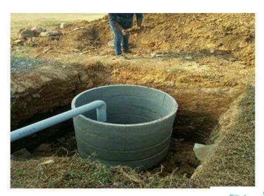
The Concrete rings were filled with stones, chips and sand to collect the rain water.
